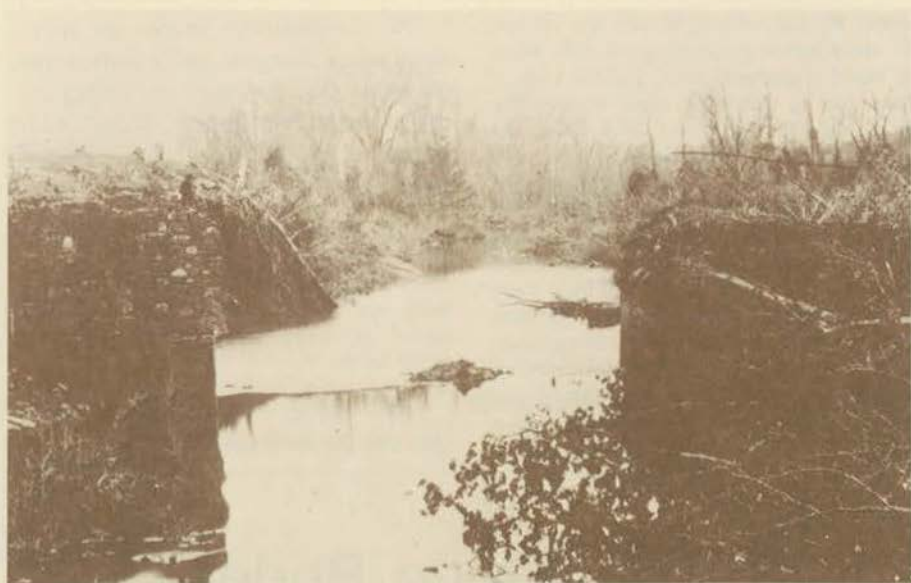
Bridge Ruins, Bull Run.
